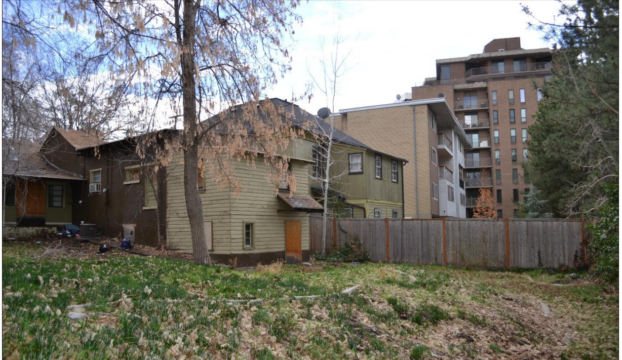
275 N. VINE STREET – REAR & SOUTHERN CONTEXT
