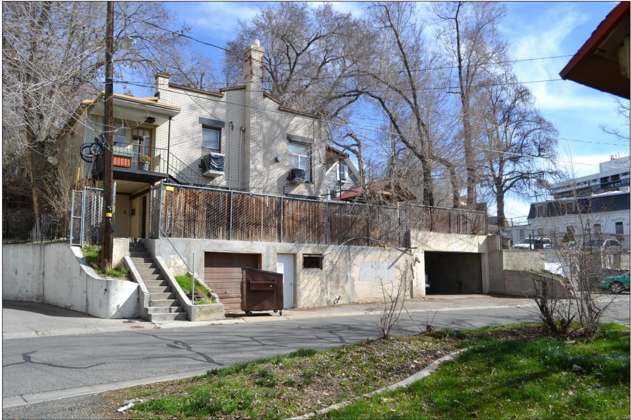
VINE STREET – FACING THE SITE
